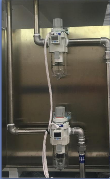
Multi-stage regulated air inlet system can effectively avoid the interference of air source pressure fluctuation
